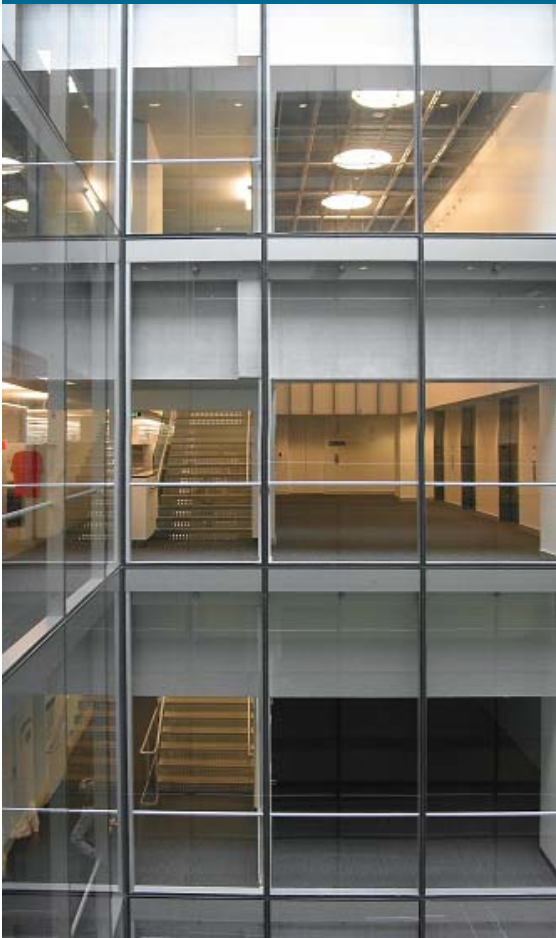
View of 7 th floor elevator lobby
