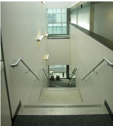
Interior of skip-stop staircase
