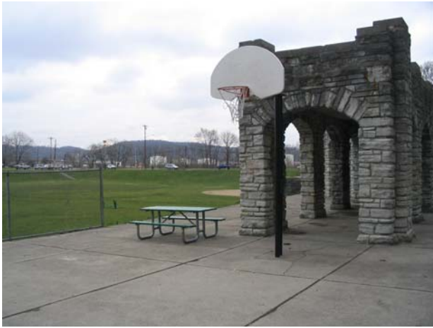
P3.1d - Condition 1 (individual cement squares are in great condition but BAD functional court condition)
