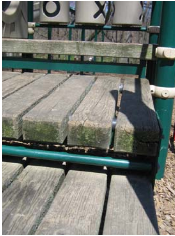
N6.3a – 3 Platforms (not a set of stairs); Condition 2 (since platform is made of wood, mold affects the function and is not considered a cleanliness issue); Cleanliness 3
