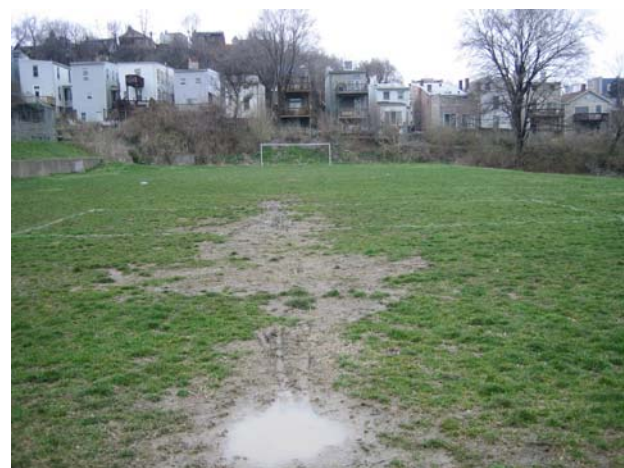
P2.3 - Drainage rating 1- water collects in middle of field.
