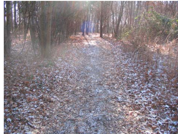
A7.4b – Unpaved Trail- Condition 3 (general form of trail can be seen and doesn't disintegrate)
