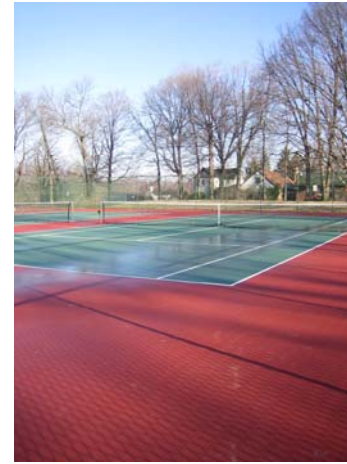
P3.1a - Court surface condition 3 (continuous surface)
