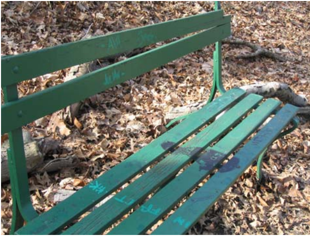
A3.5a – Places to Sit/Rest- Condition 1 (back support broken, uneven seat)
