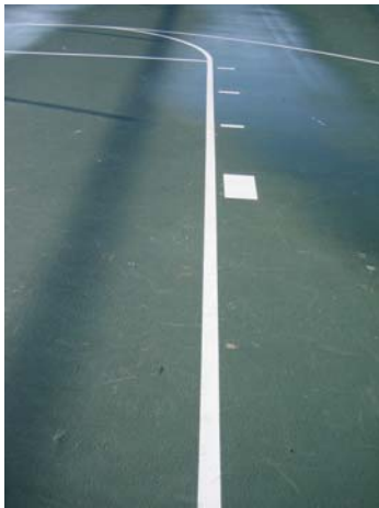
P3.5b - Striping, line condition 3
