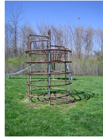
O2.2b - Jungle gym; Condition 2 (rust), Cleanliness 3
