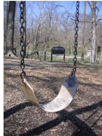
N8.3b - Swing condition 2 (rust on chains and seat is worn); Cleanliness 3
