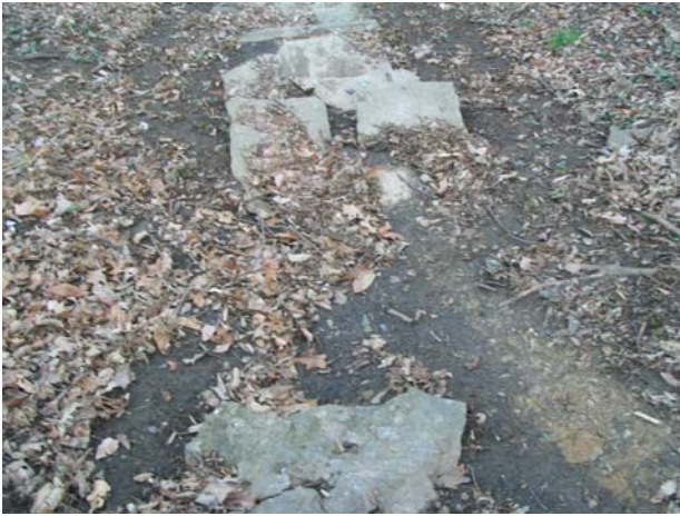
A1.4a – Paved Trail- Condition 1 (missing and broken sections)
