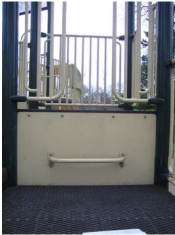
N5.1b -Functional ladder (rung), Condition 3; Cleanliness 3
