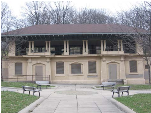
F2.1a – Shelter/Pavilion presence “yes”
