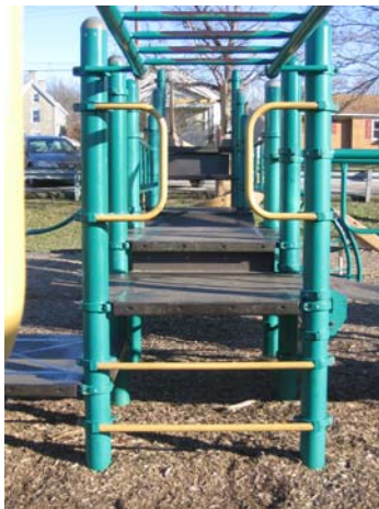
N5.2 - Do not count platforms arranged in this manner as stairs.
