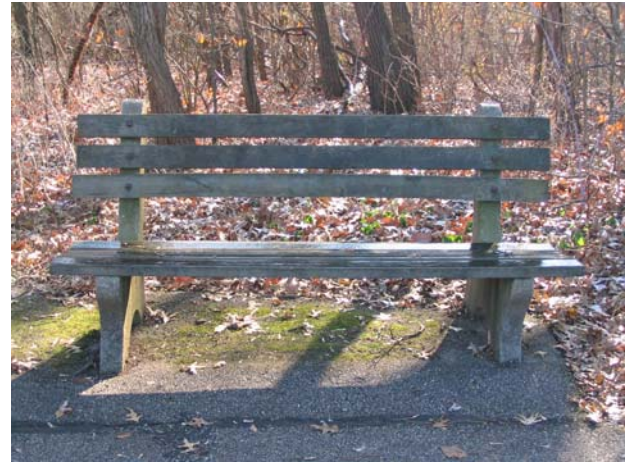
A3.5b -- Places to Sit/Rest- Condition 3 (level, proper height off ground, no missing or broken parts)
