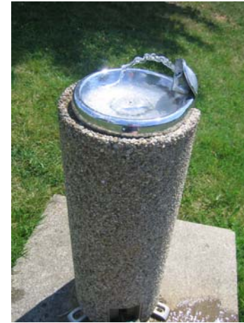
E1.4a – Condition 3 (Water flow at proper height and is contained; Water drains away.)
