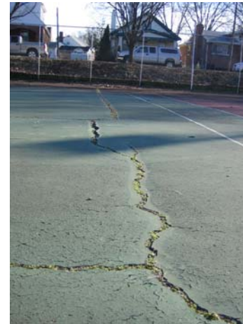
P3.1c - Court surface condition rating 1 (cracked surface, non-continuous surface)
