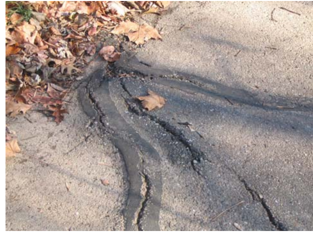
A1.4b - Paved Trail- Condition 2 (minimal amounts of patching and cracks)
