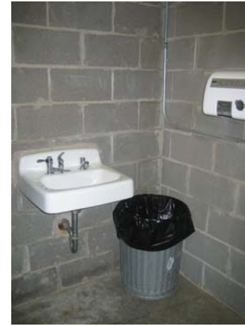
F1.4b – Cleanliness 3, Condition 3
