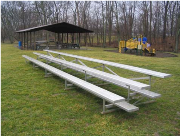
H4.1a- Metal bleachers present “yes”; Condition 3; End caps “yes”
