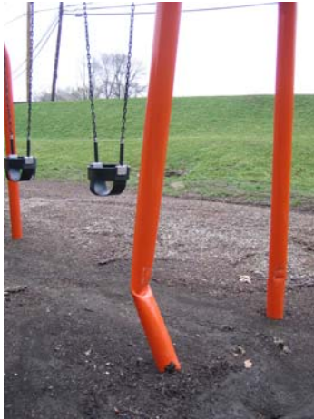
N8.3c - Swing condition 1 (not functionally safe); Poor drainage as well.
