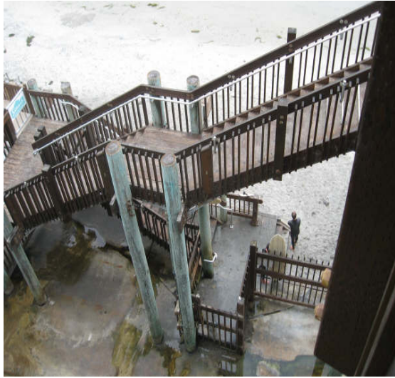
D5.3a —Accessibility “2” (stairs needed to access beach)
