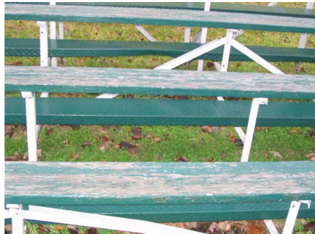
H4.3b- Bleacher Cleanliness 2 (peeling paint); Condition 3 (paint condition does not affect the bleachers’ functioning as seat).
