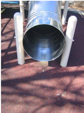
N4.11b – “Yes” Drained landing area (no bowl shape) & “Soft” landing area (rubberized surface)
