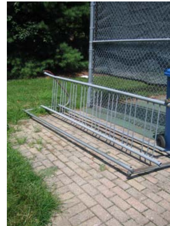
K2.1- Example of a metal bike rack; Secure to ground “no”; Lock available “no”; Covered “no”
