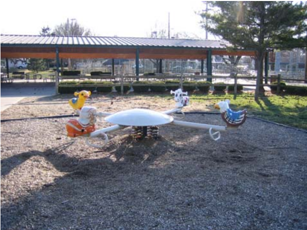
O5.7a - Spring Toy Spring Coil NOT encased
