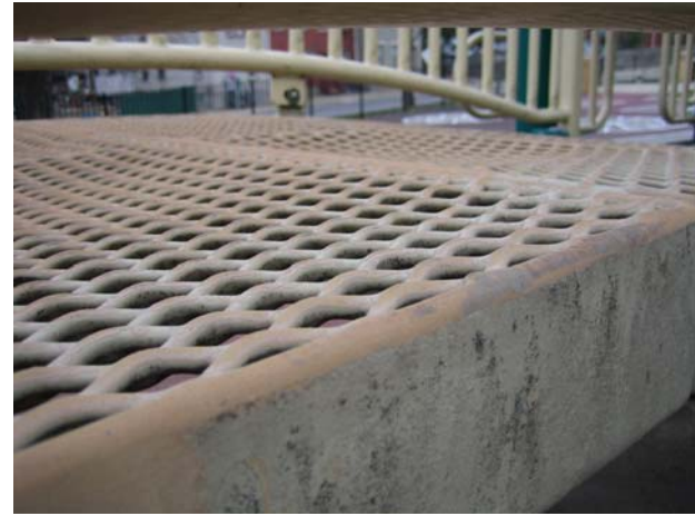
N6.3b - Platform Condition 2 (difficult to see but indentations in surface and less secure feel to touch); Cleanliness 2 (visible dirt, needs paint)
