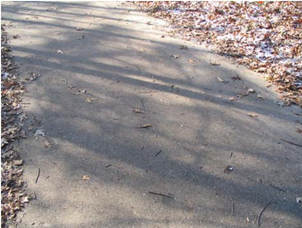
A1.4c - Paved Trail- Condition 3 (no missing/broken sections, patching, or tree roots under surface)
