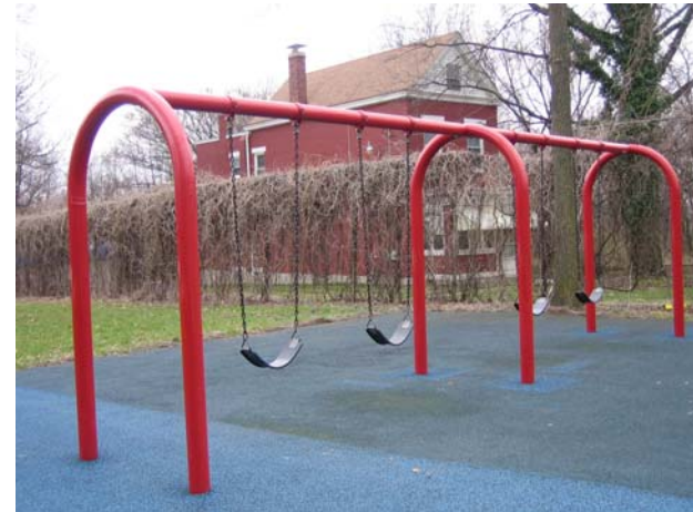
N8.10b – “Yes” drainage under swings (flat without indents or bowl shapes that allow water to pool)
