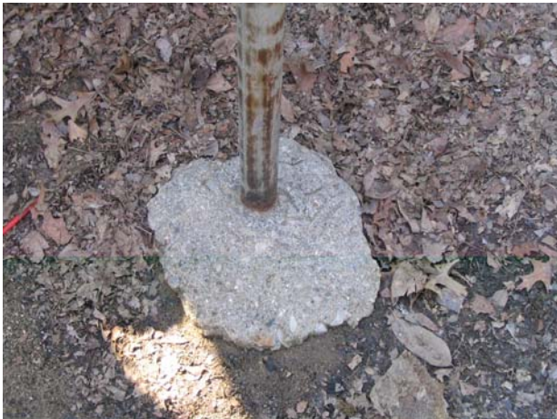
N4.3c - Base of Sliding Pole, Condition 1 (dangerous with cement base and kids potentially falling)
