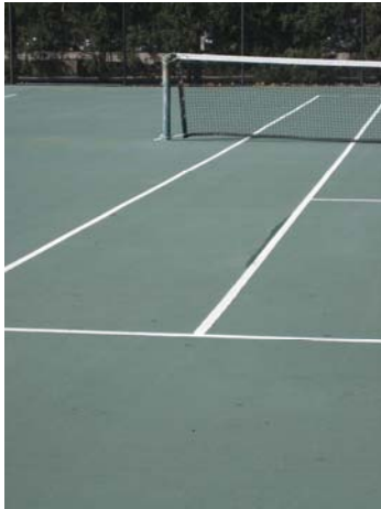
P3.1b - Court surface condition 3
