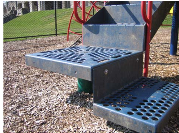
N6.2c - Not a platform; just a functional stair that is larger than the other stairs within the set.
