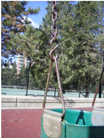
N8.3a- Swing condition 2 (due to rust)
