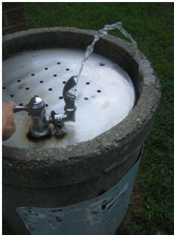
E1.4b – Condition 2 (Water flow at proper height & drains way BUT water is not contained.)
