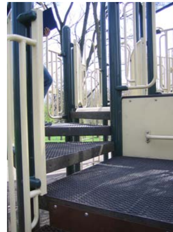
N6.2e – Rate as platforms – NOT STAIRS. Each level is counted as a platform. Platforms are often arranged in a step-like fashion, so take care in making the distinction between the two.
