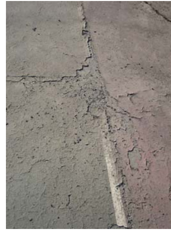
P3.5a - Striping, line condition 1
