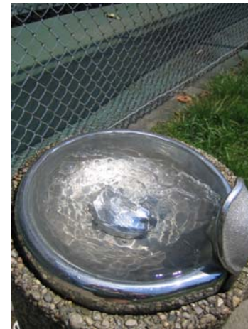
E1.4c – Condition 2 (Water pools & does not drain)
