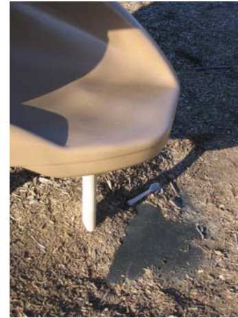
N4.11a – “No” Drained landing area & “Hard” landing area; Mulch is cleared away and slight bowl shape
