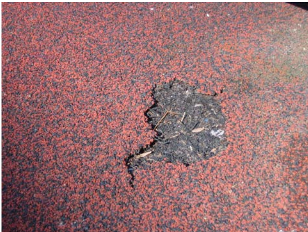
N2.2 - Ground Surface Condition 2
