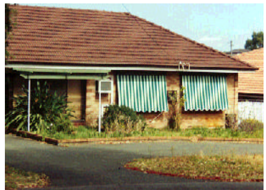
Fig. 47 Poorly maintained garden
