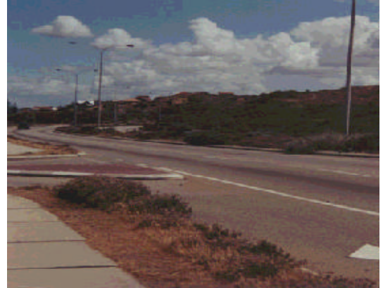
Fig. 35 Traffic island & median refuge
