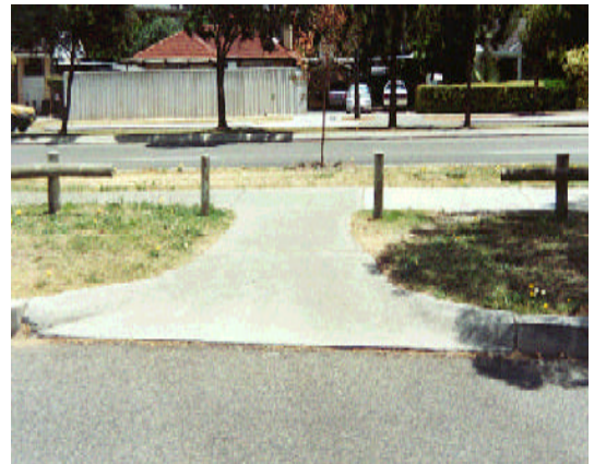
Fig. 33 Access lane for no through road
