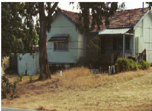
Fig. 46 Poorly maintained garden
