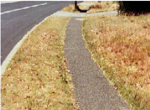
Fig. 8 Between 1 & 2m of kerb
