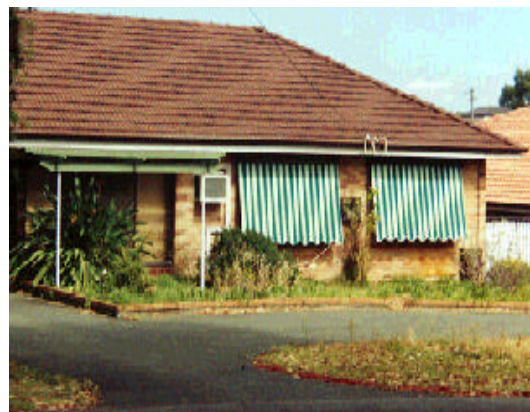
Fig. 51 Poorly maintained verge
