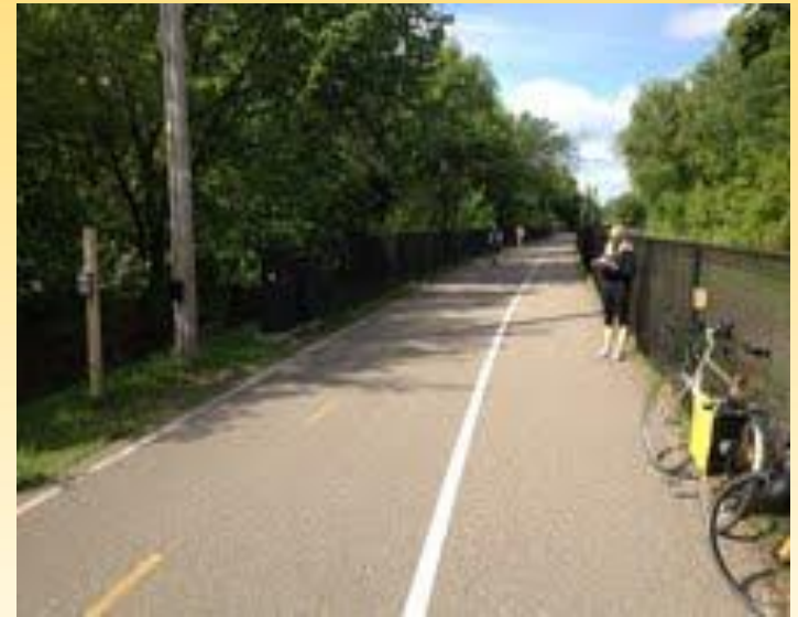
Typical Monitoring Site: Midtown Greenway
