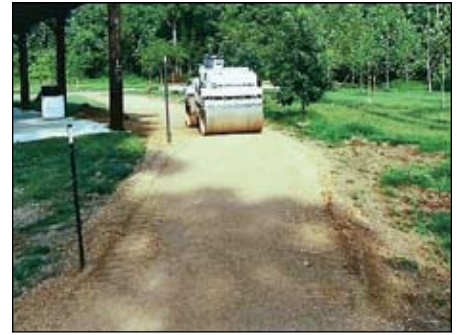
Workers build the McKenzie Creek Trail in Piedmont, MO.
