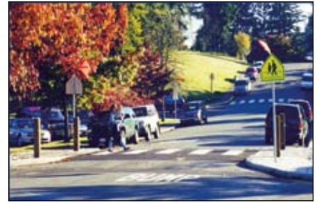
A raised crosswalk and curb extensions at a school crossing in Bellevue, WA.
