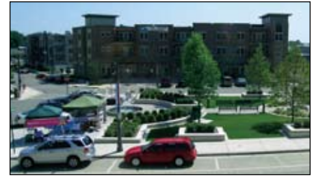
Cannery Square in Sun Prairie, WI: The result of a traditional neighborhood development ordinance that supports active living for residents.
