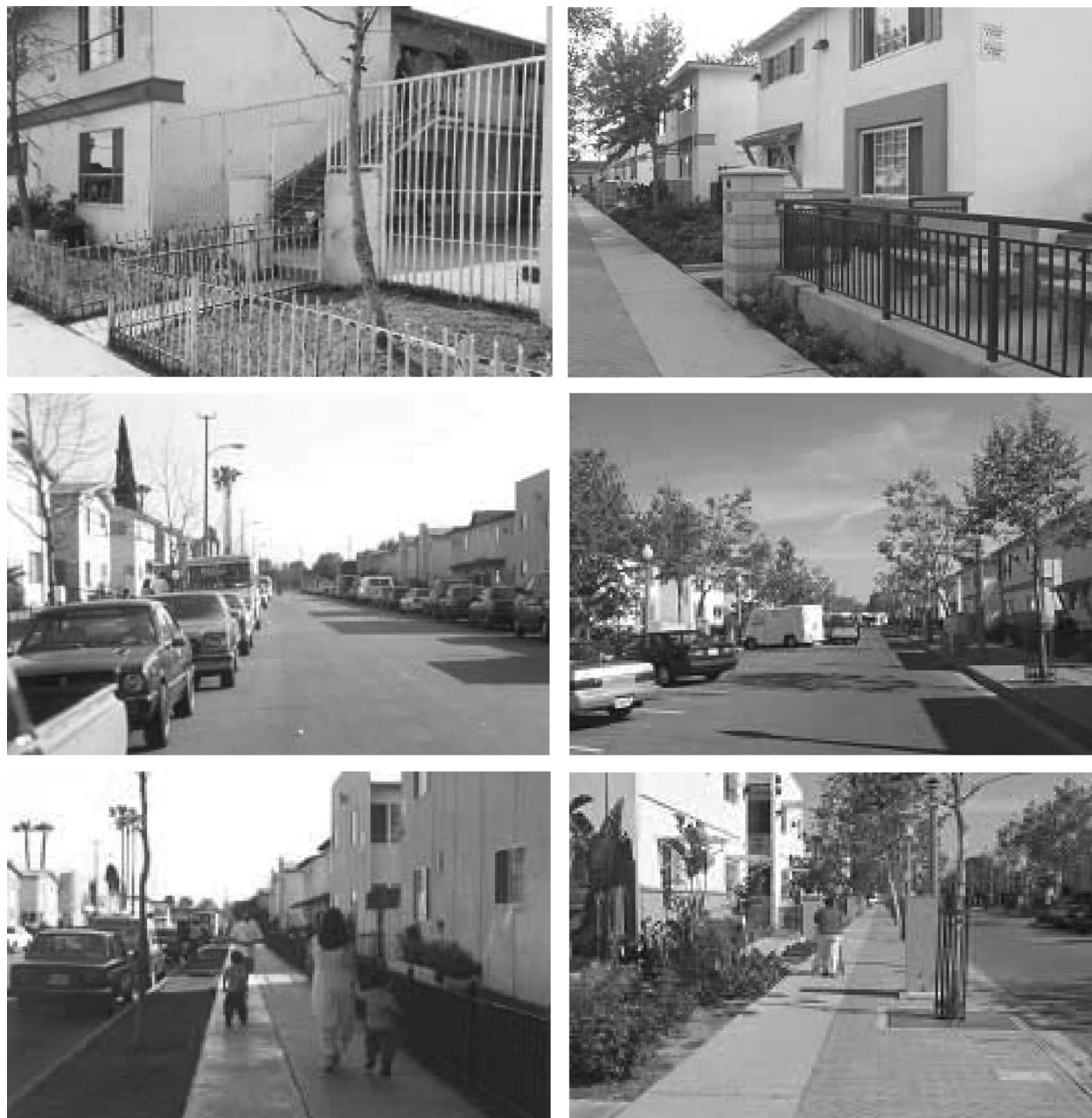
Figure 1. Minnie Street before (left) and after (right) renovation.
