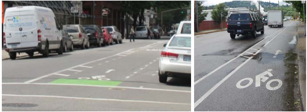
Figure 2 Buffered Bike Lanes, Portland, Oregon.
