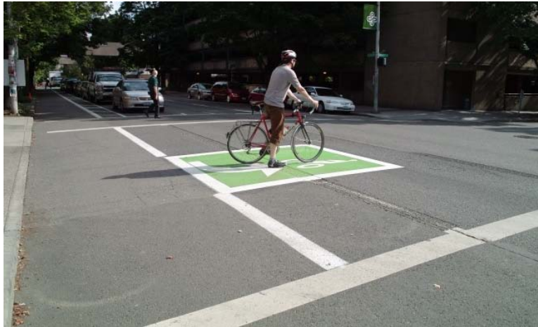
Figure 13 Two-stage turn queue box. Portland, Oregon.
