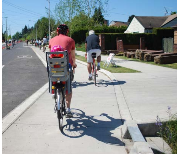
Figure 26 Raised Cycle Track, NE Cully Blvd., Portland, OR.
