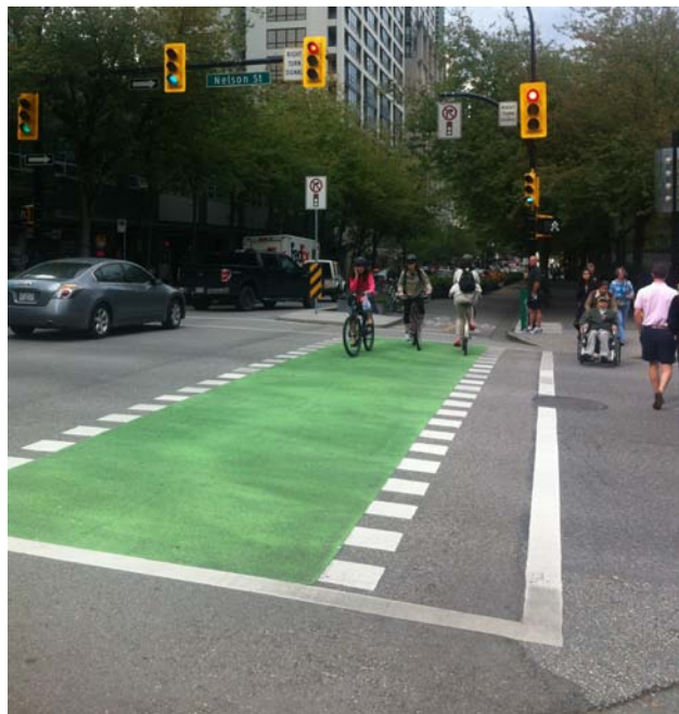
Figure 12 Bicycle Crossing Marking, Vancouver, British Columbia.
