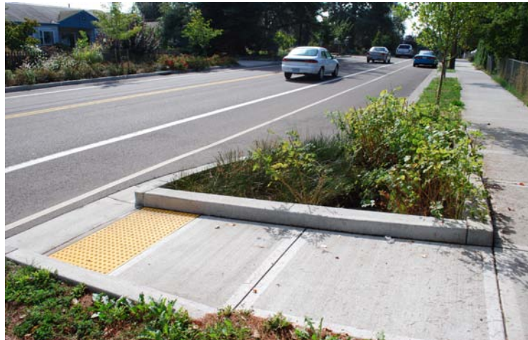
Figure 15 "Green" Curb Extension with storm water capture. Portland, Oregon
