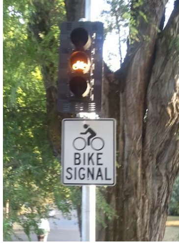
Figure 18 Bicycle Signal Head, Portland, Oregon.
