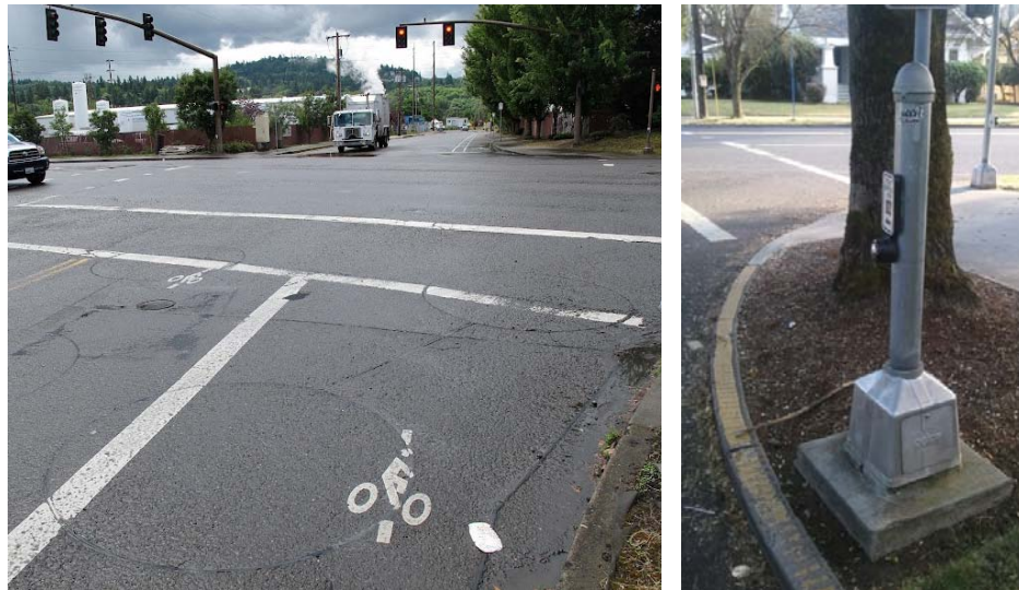
Figure 20 Bicycle Loop Detection and Bicycle Push Button Detection, Portland, Oregon
